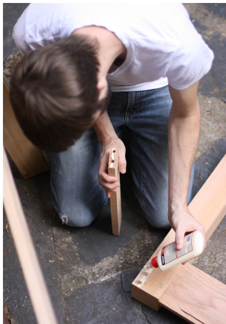
I used dowels and wood glue to join the aprons with the legs
